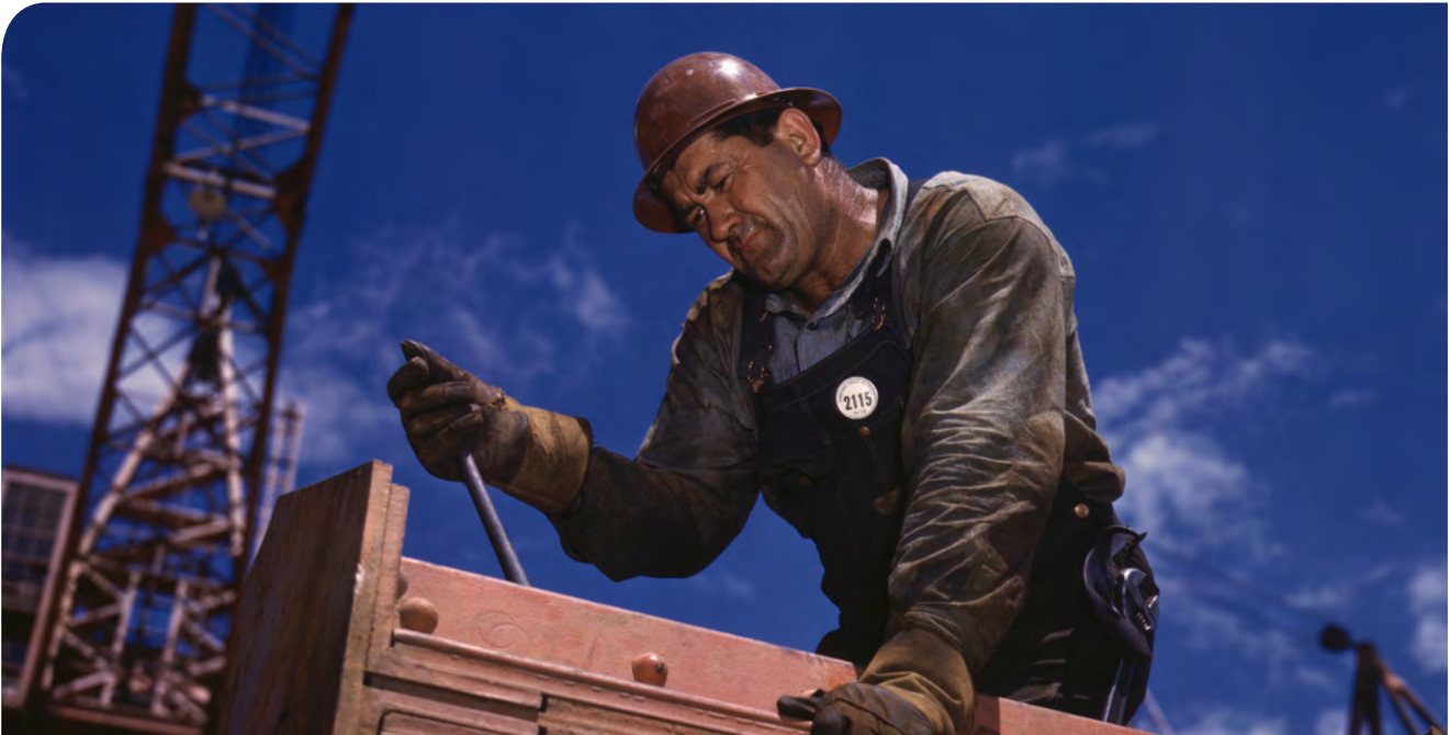
Photo 4: Rigger at work Credit: Alfred Palmer
